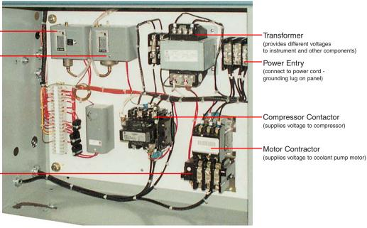
Refrigerant High Pressure Limit - (protects from excessive condensing pressures)
