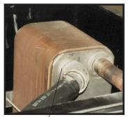
Typical hot gas bypass valve Figure 6.2H
