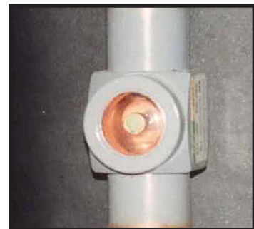
Refrigerant sight glass Figure 6.2E
