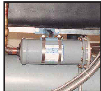
Typical filter-drier Figure 6.2D
