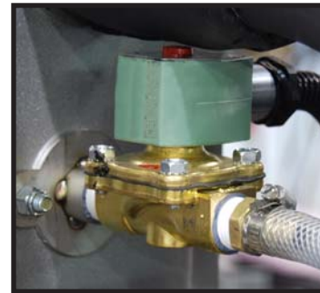
Make-up solenoid valve
