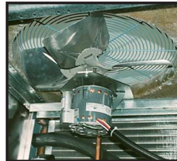
Typical fan assembly
