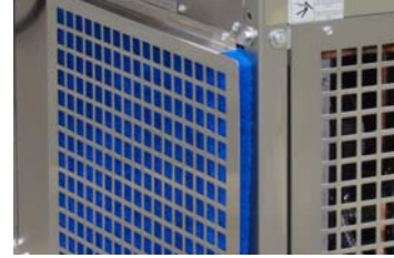
Typical Condenser Screen.
