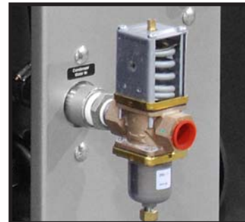
Typical water saver regulator valve.
