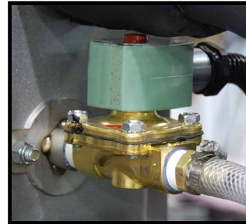
Make-up solenoid valve
