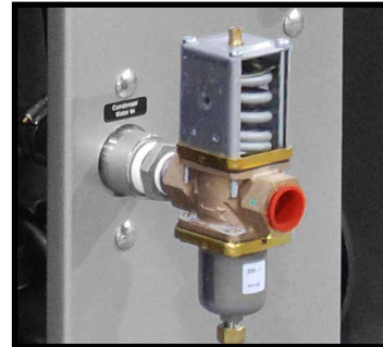
Typical water saver regulator valve.
