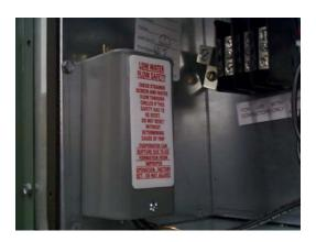
Generally the cause will be low or insufficient water flow caused by a clogged "Y" strainer or restricted flow in the process. This safety can also be tripped by low ambient conditions overnight or during shipping. Resetting this control and not determining the cause for tripping can cause the evaporator to freeze and rupture.
