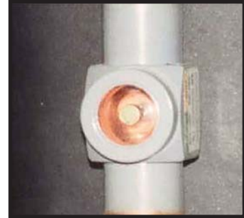
Refrigerant sight glass Figure 6.2D
