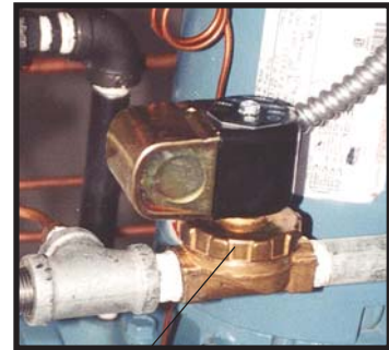
Make-up solenoid valve
