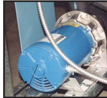
Pump Motor Assembly Figure 6.1A
