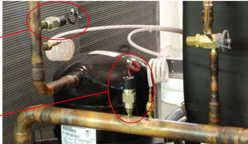
Typical placement of non-adjustable "fixed" pressure switches.
