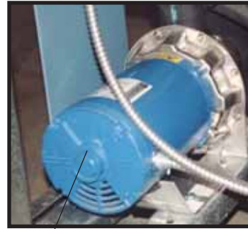
Pump Motor Assembly Figure 7.1A
