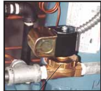
Make-up solenoid valve
