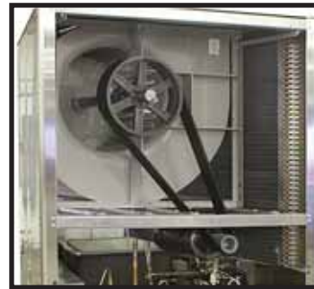
Typical blower assembly Figure 3.4B
