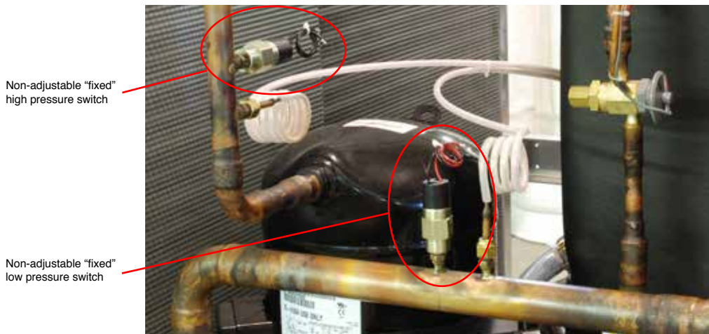
Typical placement of non-adjustable "fixed" pressure switches.
