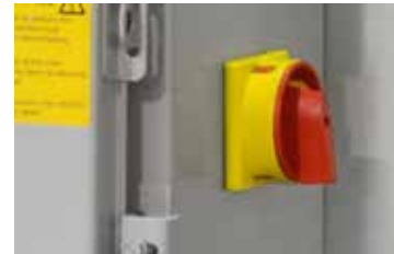
Non-fused disconnect switch.
