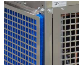
Typical Condenser Screen.
