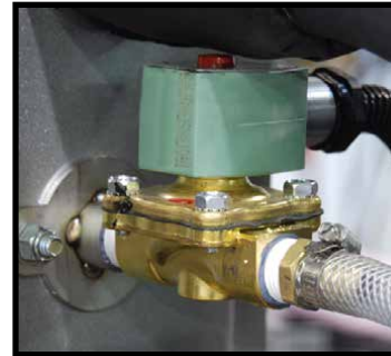
Make-up solenoid valve
