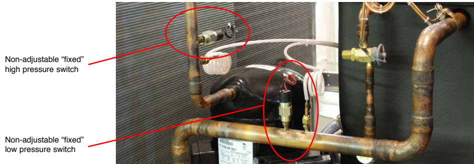
Typical placement of non-adjustable "fixed" pressure switches.
