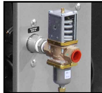
Typical water saver regulator valve.
